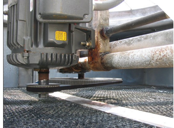
After: Same unit with synchronous belt drive.
