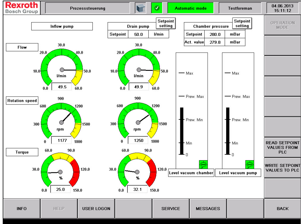
Fig. 18: PROCESS CONTROL screen
