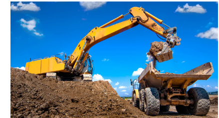
Off Road Construction
